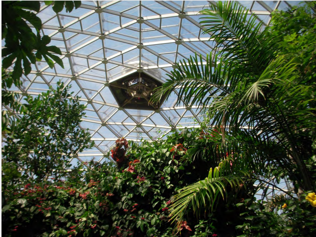
Figure 1. The roof of the Climatron ®, a geodesic glasshouse hosting tropical collections at Missouri Botanic Garden
