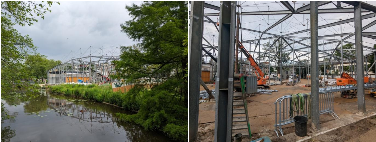
The empty frame of the Conservatory under restoration
