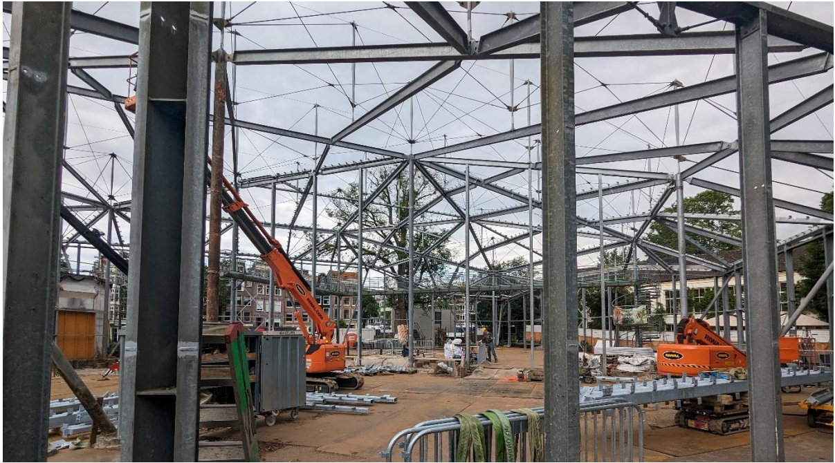
The main display glasshouse in Amsterdam is being renovated.
