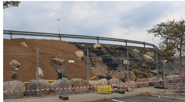
Figure 37 stop 2, top layer and under layer of substrate
