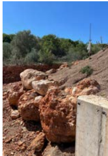
The substrate under the gravel
