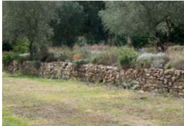
The dry stone walls with drains behind
