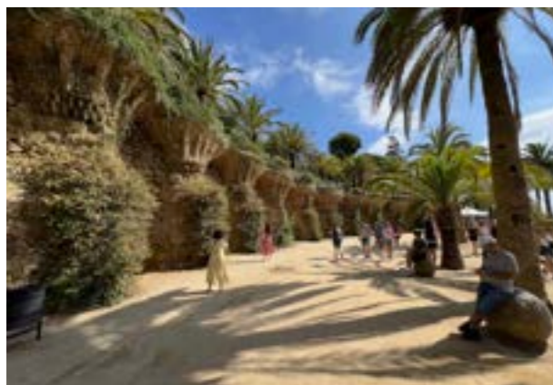
Pillars on the level above the plaça with Bougainvillea glabra growing up them
