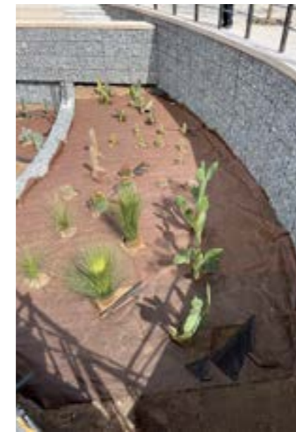
Cacti garden down to the new tram stop
