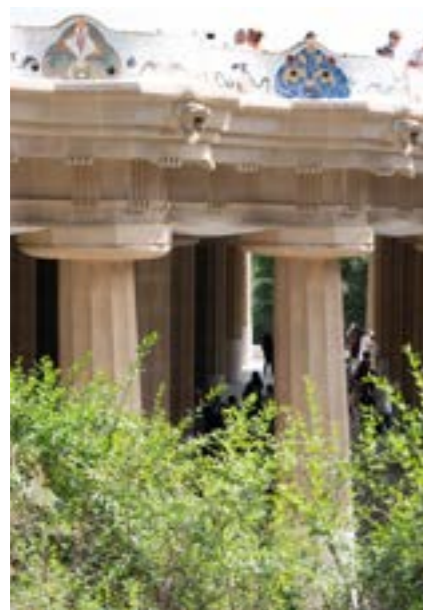
The columns water flows through underneath the plaça
