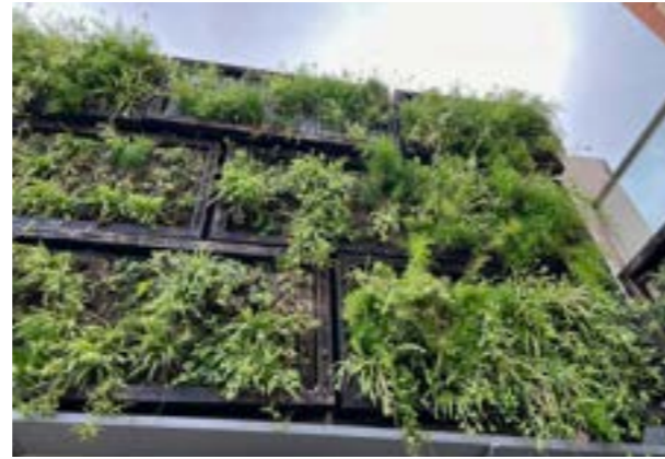
Packed earth on the lower section and metal cage on the top section
