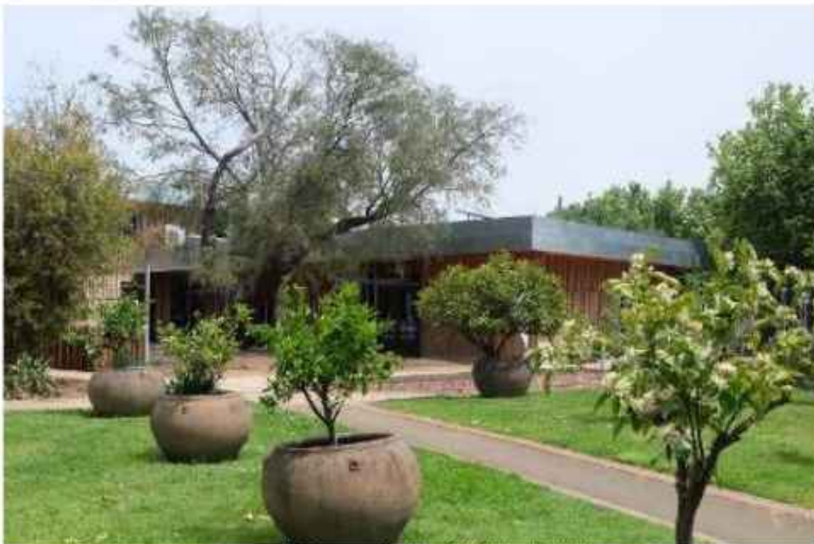
Entrance to the St Kilda Building
