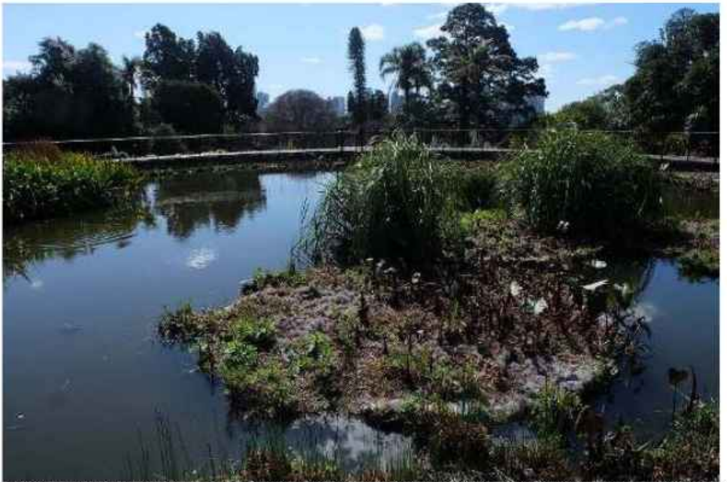
Floating islands move across the top of Guilfoyle's Volcano reservoir, softening the edges of the historic bluestone. These vegetated platforms contribute to water filtration, create habitat, and add movement to what was once purely functional infrastructure, demonstrating how heritage structures can be ecologically reimaged.
