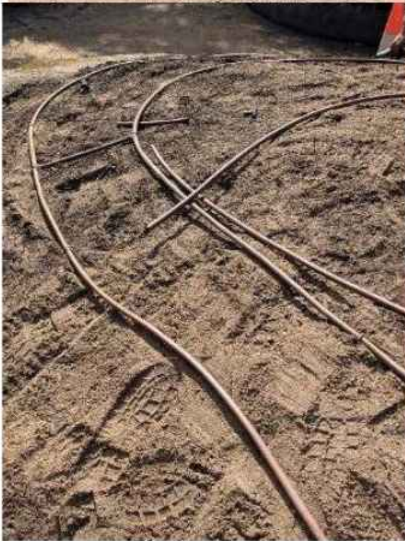
Irrigation Installation – Grey Colour Garden The staged process of installing irrigation within the grey-toned section of the Colour Specification Garden. Tubes were connected, tested, and faults identified before being backfilled with soil and planted
