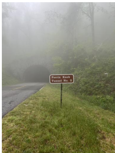
Fig. 1 Ferrin Knob Tunnel No.2
